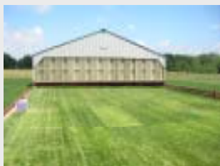
Figure 1. Rainout shelter (180 m 2 ) at Rocky Ford Turfgrass Research Center near Manhattan, KS. The rainout shelter automatically moved over plots (on tracks) when rainfall began, then retracted one hour after rainfall ended.
