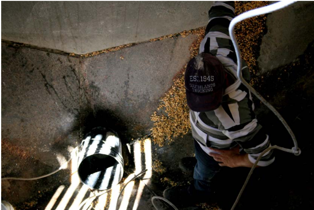
A worker waits for instructions on what to do at the bottom of the broken grain bin. The corn is what is stored in the bin they are trying to fix. Water had gotten into the bottom of the tank from the rains a couple days ago.
