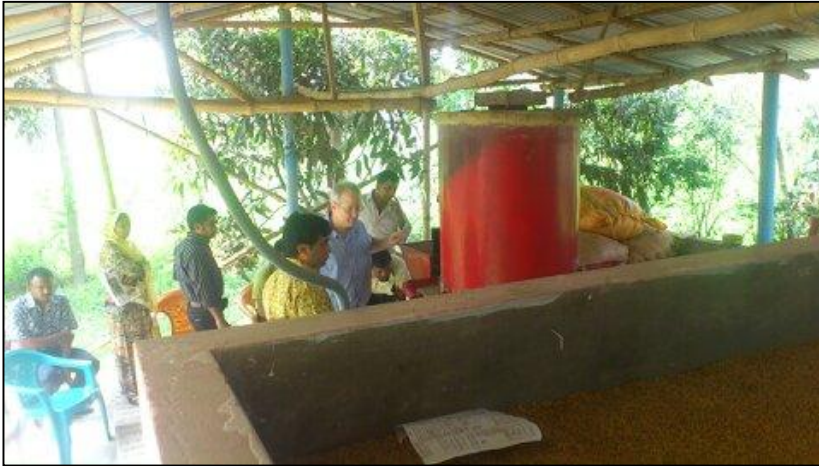
Photo 1: Examining furnace and cyclonic cleaner
