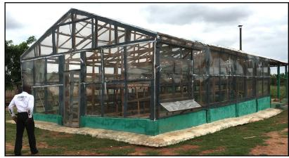
To address this problem, the PHLIL Ghana team, led by a young engineer at the Kwame Nkrumah University of Science and Technology (KNUST) in Kumasi, Ghana, developed the solar biomass hybrid dryer. Based on initial assessments, the team identified the greatest potential for impact at the market and meso level and so designed this dryer to be built at market centers or at larger producers.
