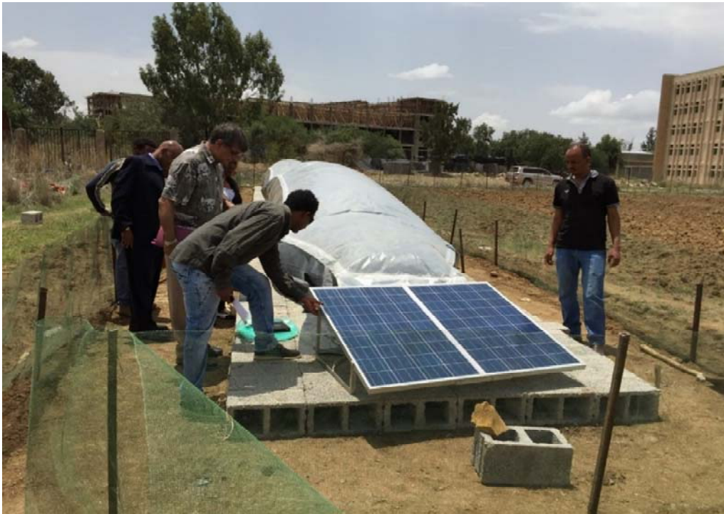
Figure 1. Members of the Feed the Future Reduction of Post-Harvest Innovation Lab Team installing a Solar Bubble Dryer (GrainPro®, USA) in Ethiopia.
