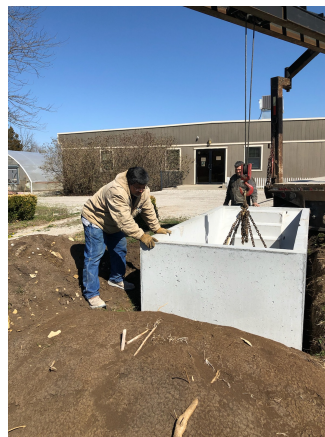
Bottom half of shelter is set.
