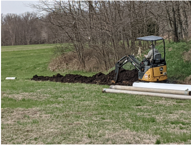
Farm crew trenches water lines.
