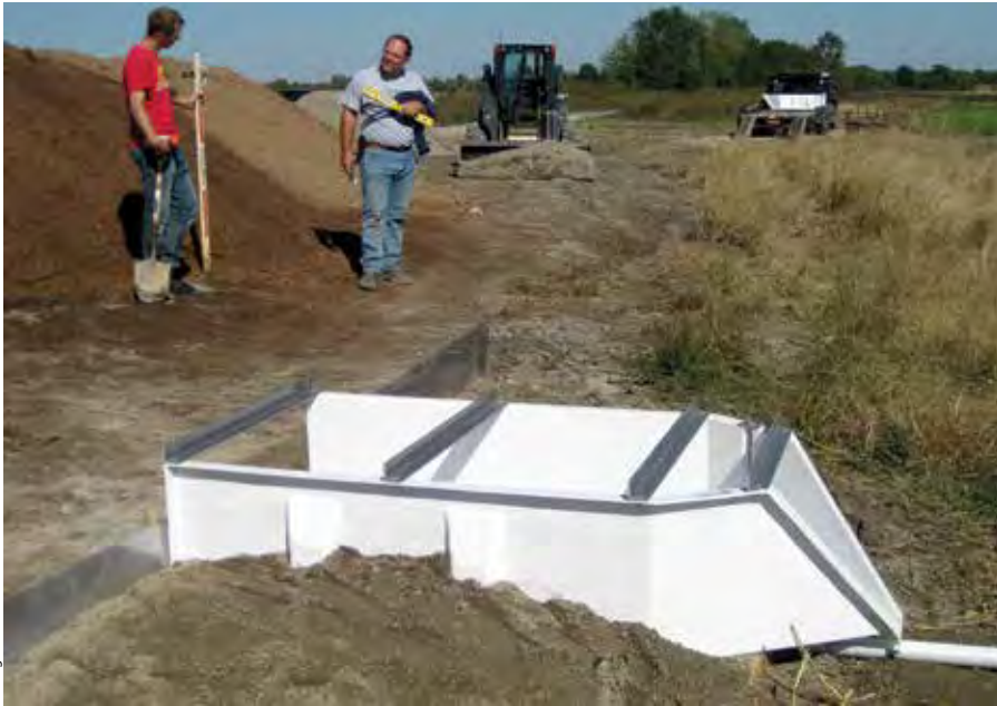
Agronomist Peter Tomlinson (right) and Barrett Smith, agronomy master's student, discuss the next step to install the flume, which captures water runoff from poultry litter.
