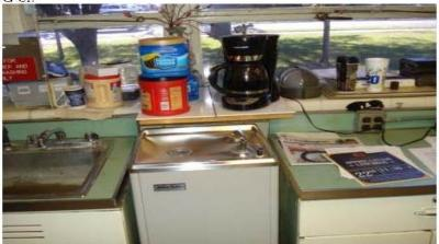
Condition: Duplex outlet within 6' of a wet bar sink was not protected by a ground fault dirouit interrupter (GFCI) outlet.
