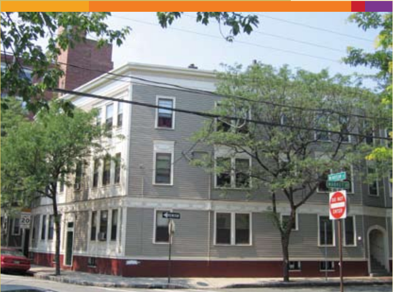
Homeowner’s Rehab, Inc. acquired, renovated, and preserved the affordability of 95 family-sized rental units scattered throughout the Wellington/Harrington and Area IV neighborhoods, including this 9-unit apartment building which was renovated in 2002.
