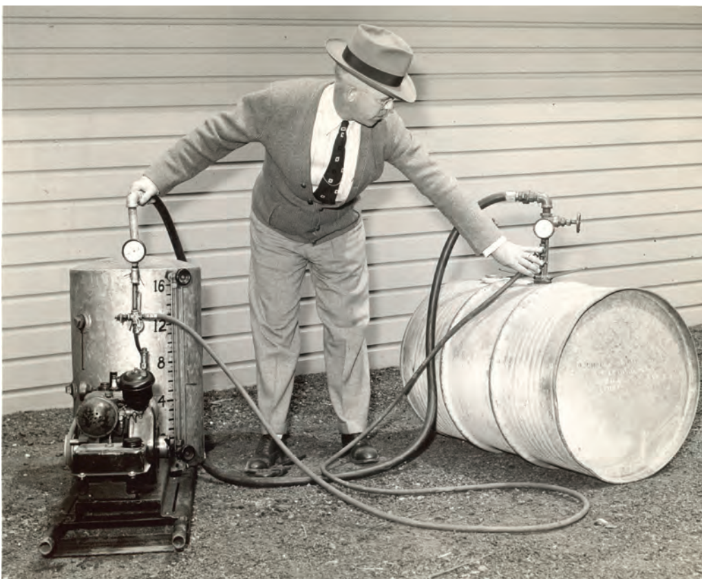
A May 1942 photo of USDA entomologist H.H. Walden demonstrating the fumigation of stored grain by means of a power compressor. The fumigation tank was filled with fumigant from a supply drum.
