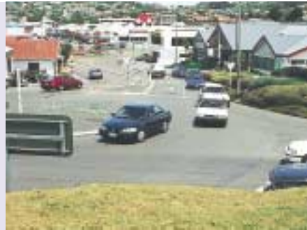
Multi-lane roundabout providing no guidance to motorists in the circulating roadway
