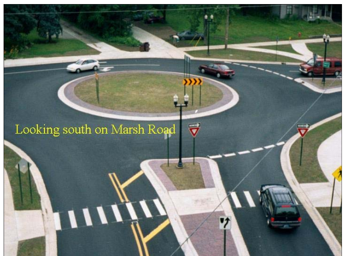
Figure 6. Okemos: Looking Southbound (Photo courtesy Ingham County Road Commission)
