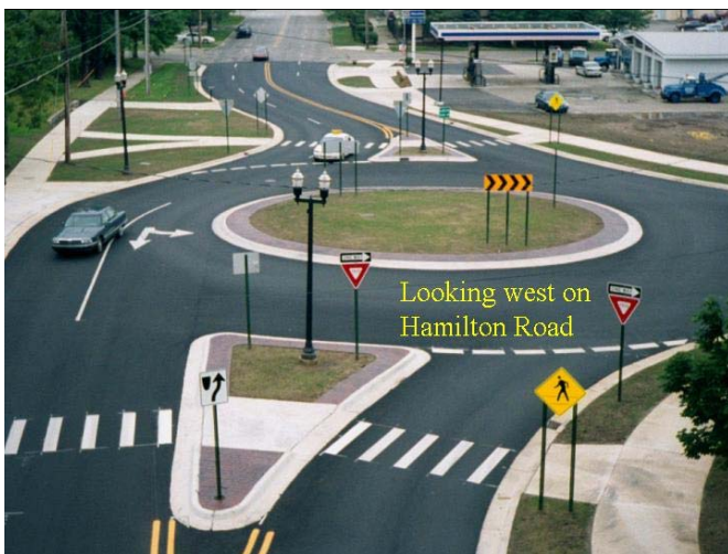
Figure 5. Okemos: Looking Westbound (Photo courtesy Ingham County Road Commission)
