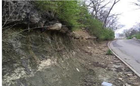
smaller shale and soil particles are washed away and the limestone is thus broken off by gravity.
