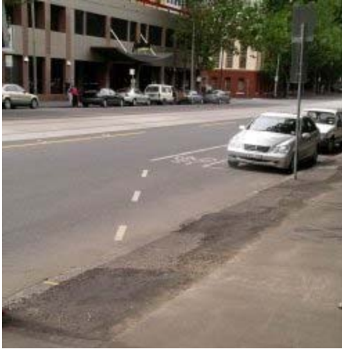
Figure 9: Curb cut approach to diverting road traffic to a multi-use path (Source: Melbourne Bicycle User Group 2005).
