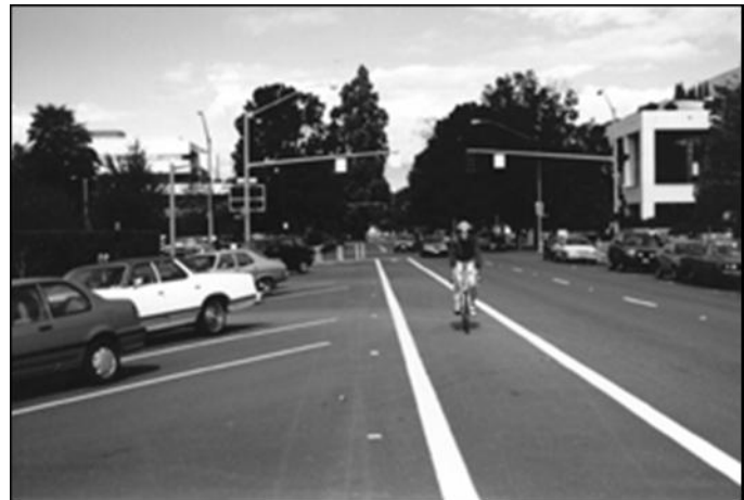
Figure 5: Bike lane adjacent to diagonal parking stalls with additional buffer zone.
