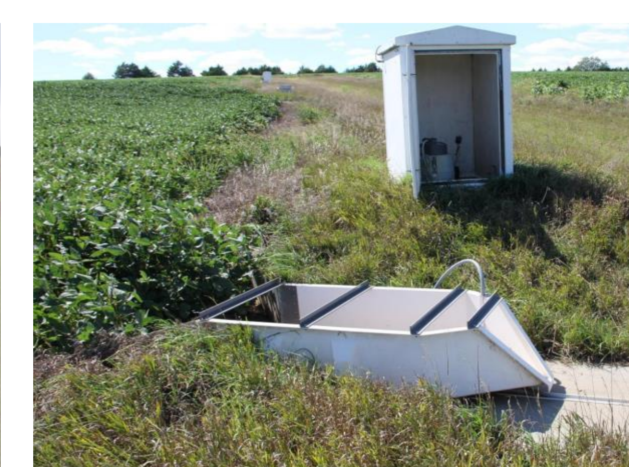
H-flume and automated water sampler shelter
