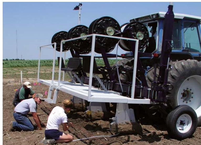
Subsurface drip irrigation tubing is installed at Kansas State University, Colby, Kan.
