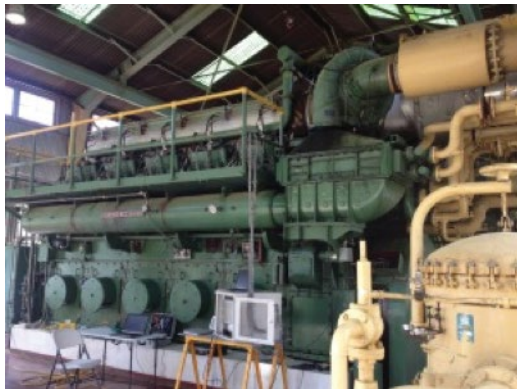
Pipeline compression engine (Source: CTS, Combined Technology Solutions)
