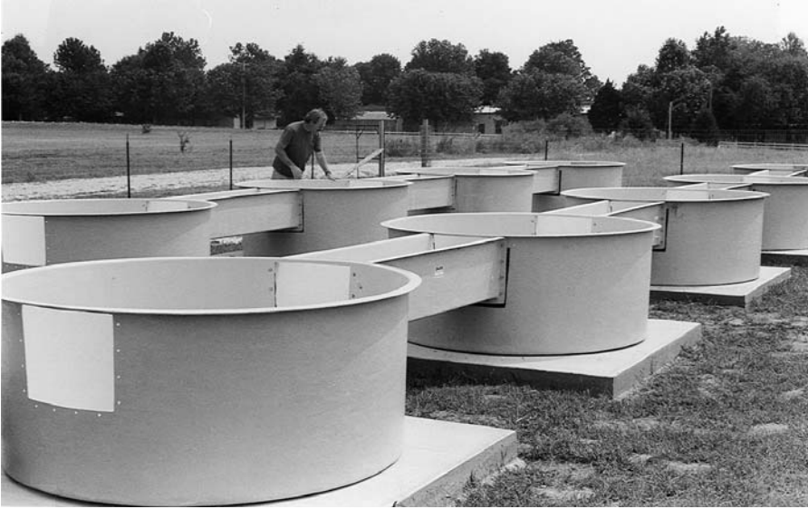
FIGURE 1.—Photograph of the original modular experimental stream system under construction at the University of Oklahoma Biological Station showing alternating pool and riffle units; one end is open to show point of attachment for the next riffle unit. Concrete pads were poured with an overall allowable tolerance of only 0.25-in difference in height to assure uniform control of water level in all units. Plexiglas observation ports had not yet been added to pool units.
