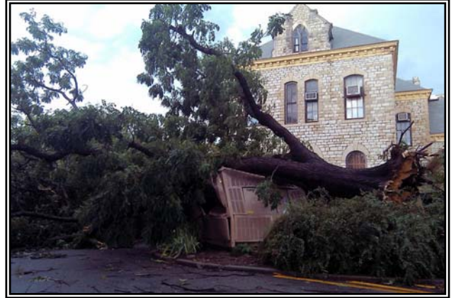
Above: A tree behind Anderson Hall broken off and lying on the chiller.
