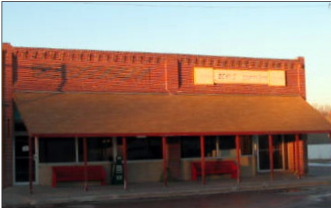
The Morland grocery store in its beginning redevelopment stages.
