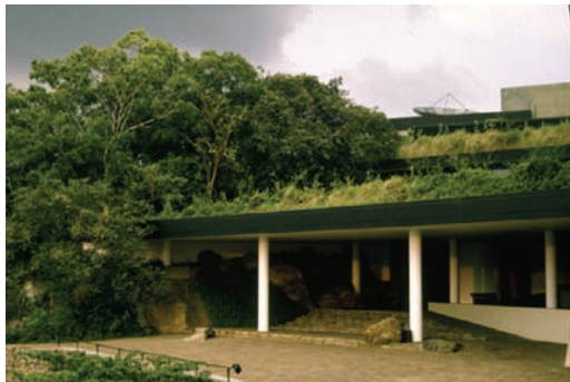
Figure 16) Hotel entrance - Use of green roofs that help cooling and contribute to environmental image.
