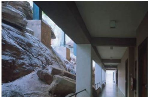
Figure 9) View along corridor dug through rock, with a wall left exposed
